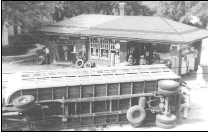
A Kleinhenz stock truck overturned in front of The Lone Pine Gas Station while rounding the corner of North Main and Pearl Streets (then Route 66). This is thought to have happened in the summer of 1944. This was the driver's last run before going into the service.
